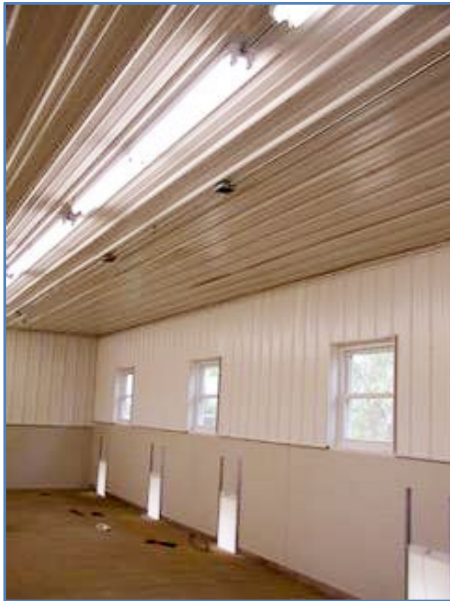
East interior wall with lighting, windows and framing for guillotine doors
